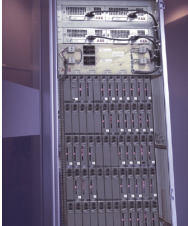
Figure 2. Harmony Rack Modules
